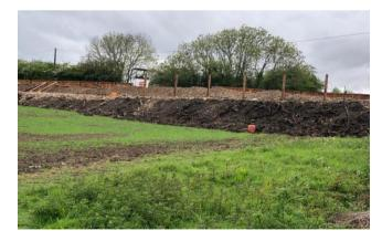
During the enlargement and levelling of the site substantial amounts of material were deposited on the ground and a large bund was constructed. There evidence no that these is groundworks were carried out in a controlled manner using approved materials or that the drainage and installation of the cesspit was approved by Building Control Inspectors
