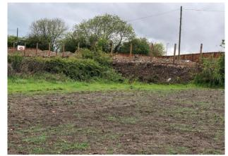
There is anecdotal evidence that vegetation from the grubbed out hedgerow and other refuse was used in the construction of the bund which may not provide a sound base for residential structures.
