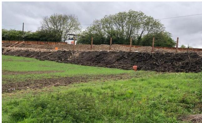
During the enlargement and levelling of the site substantial amounts of material were deposited on the ground and a large bund was constructed. There is no evidence that these groundworks were carried out in a controlled manner using approved materials or that the drainage and installation of the cesspit was approved by Building Control Inspectors
