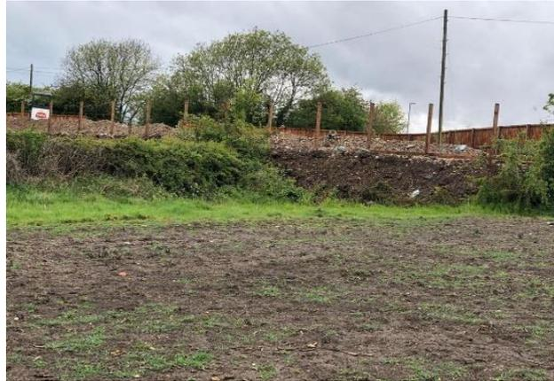
There is anecdotal evidence that vegetation from the grubbed out hedgerow and other refuse was used in the construction of the bund which may not provide a sound base for residential structures.
