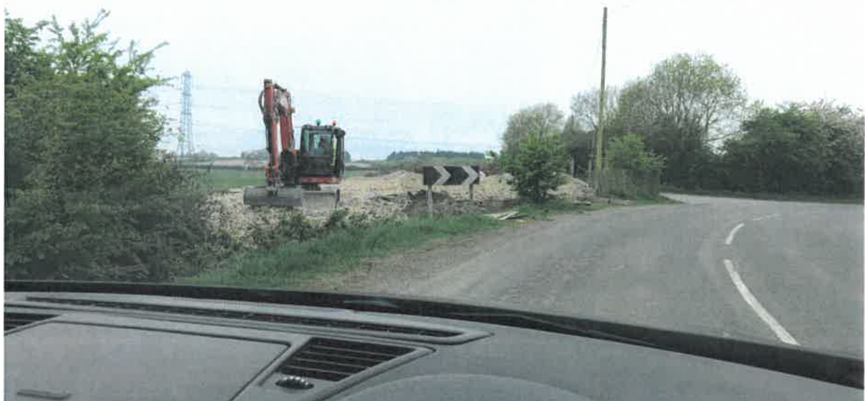
View exiting Broughton on Northampton Road with groundworks underway to remove hedging and prepare surface with hardcore. We are assuming this is for a new service road to the Old Willows plot as per the red line Location Plan but no detail has been provided within the application. Views through to the open countryside should be visible here.
