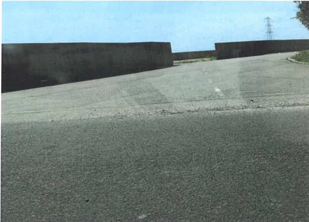
View of reconfigured site entrance entering from Northampton Road from the A43
